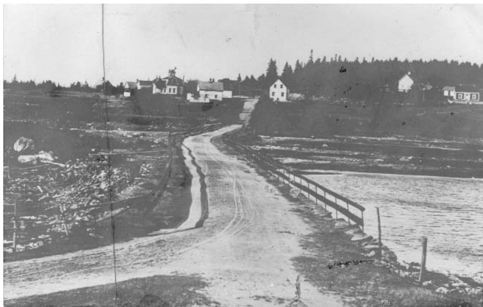
Charlotte Ricker captions this photograph as follows, "The lower dyke, Glenwood, with the 'Corner', and the main road, in the distance. The building in the centre is a store". ATCHA Photo#P2006:574.
